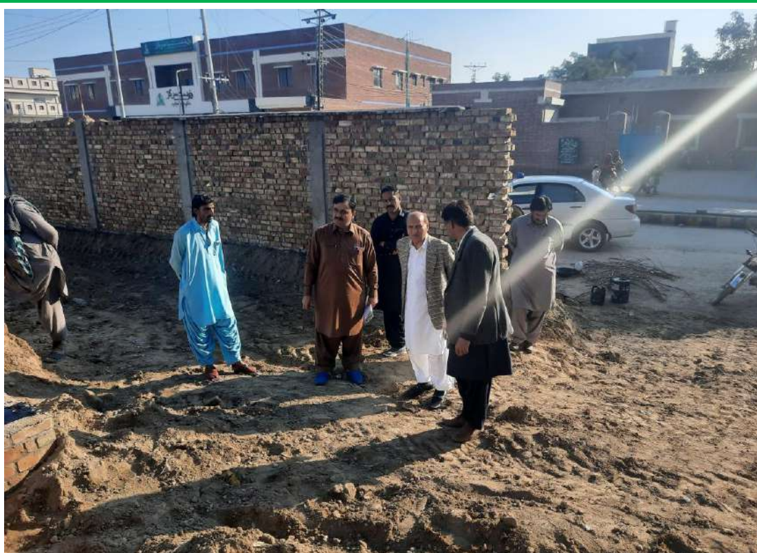
Construction of Regional Office Dera Ghazi Khan
