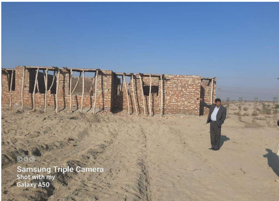
Construction of Regional Office Muzaffargarh
