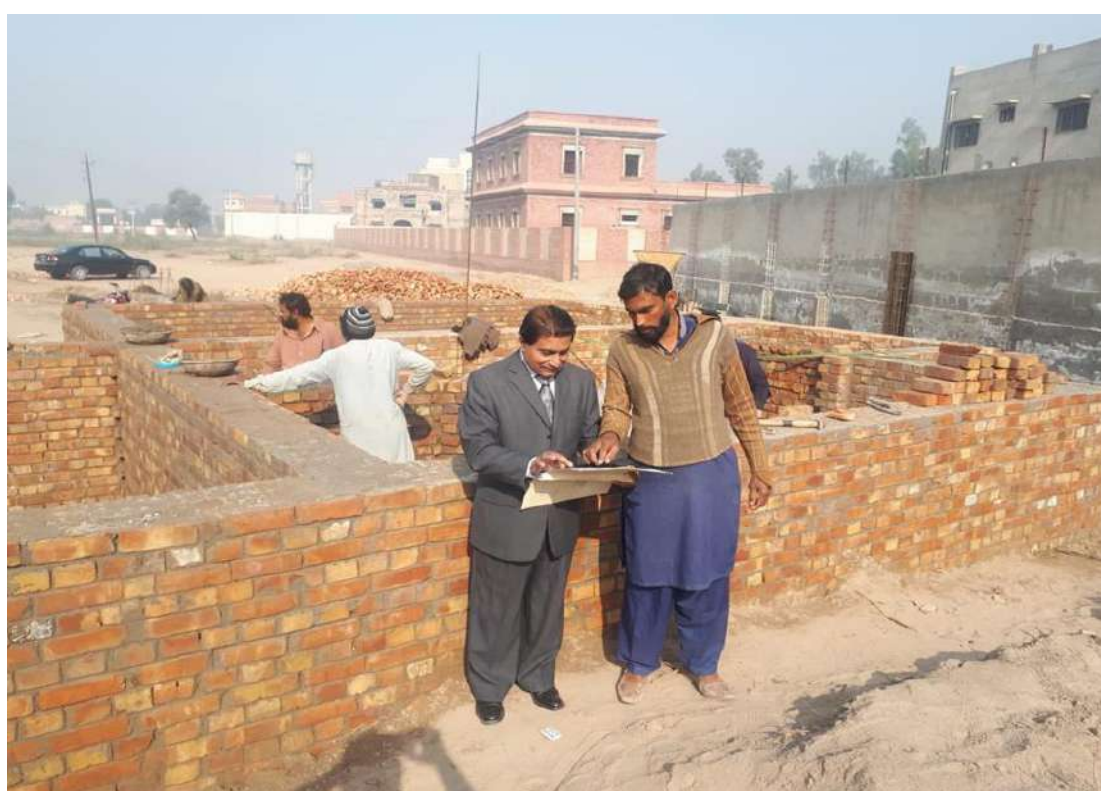
Construction of Regional Office Jhang
