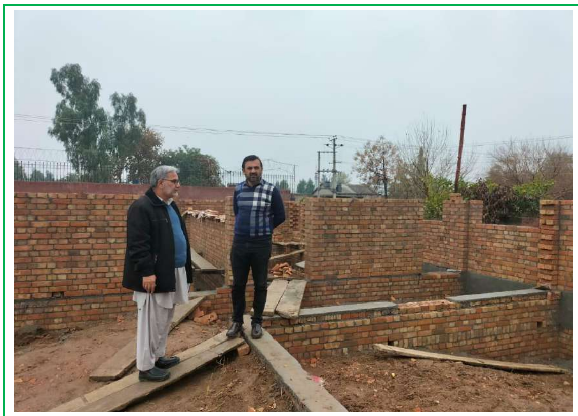
Construction of Regional Office Mianwali
