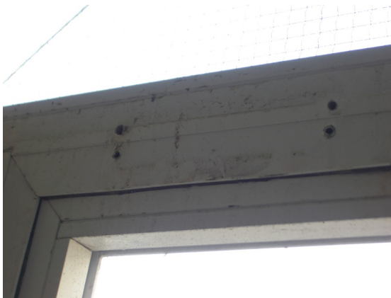
3: Upper section of the Door on which the door closing mechanism was positioned.
