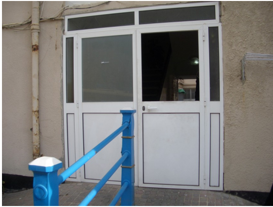
1: Doorway, being access to the Building, showing section where pane needs to be replaced.
