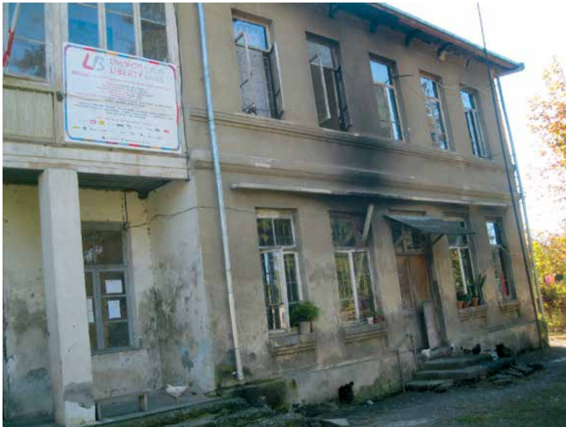
Orsantia Municipality Building
