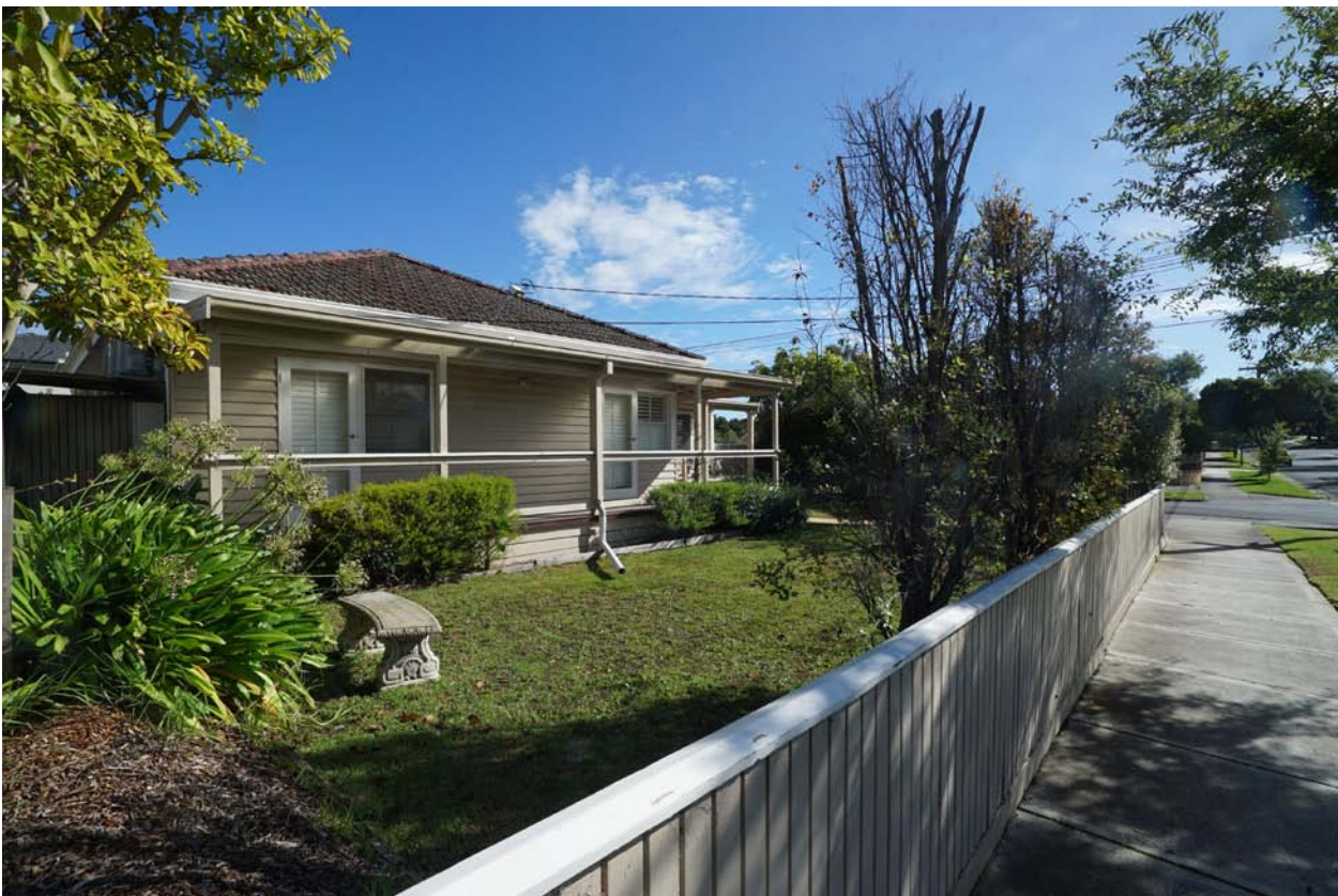
Figure 2: Photograph of temporary pipework at Mr Wilson's house
