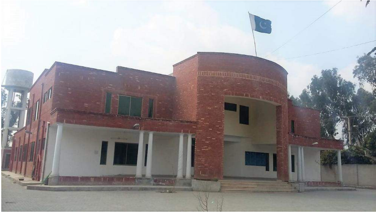
Front elevation of newly constructed building of Regional Office Sargodha
