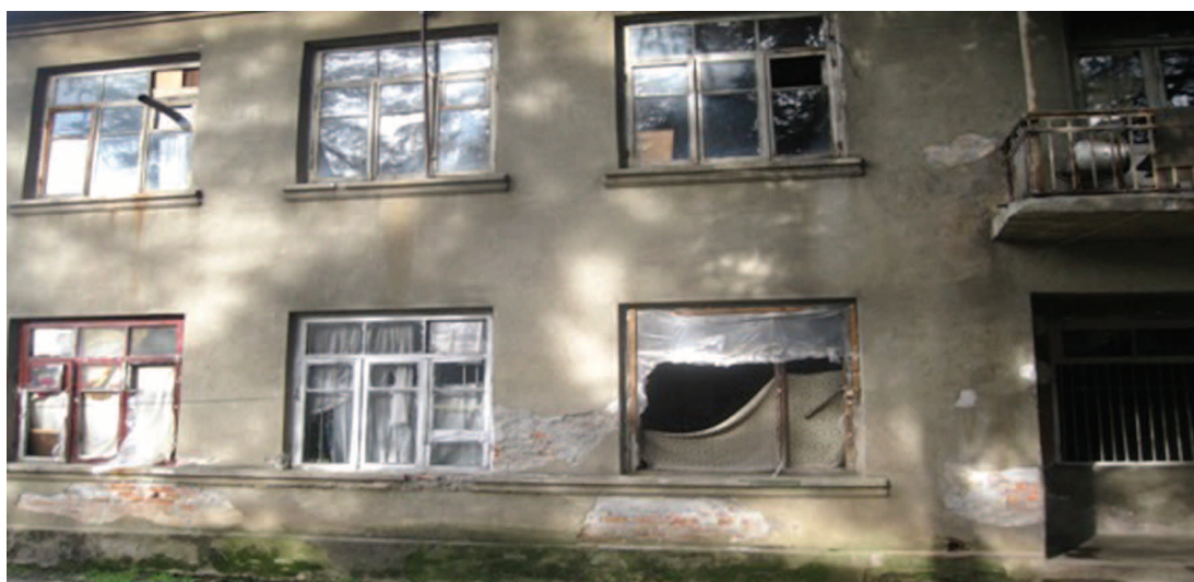
Zugdidi regional hospital building.
