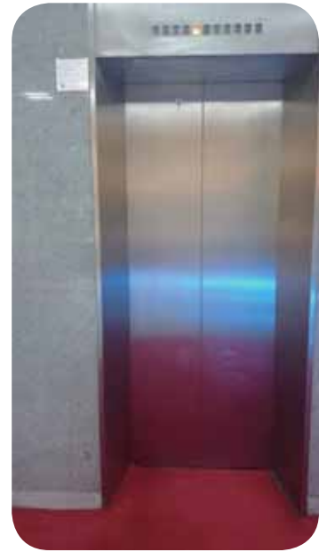
CY proposed corrective measures to ensure safe elevator use
